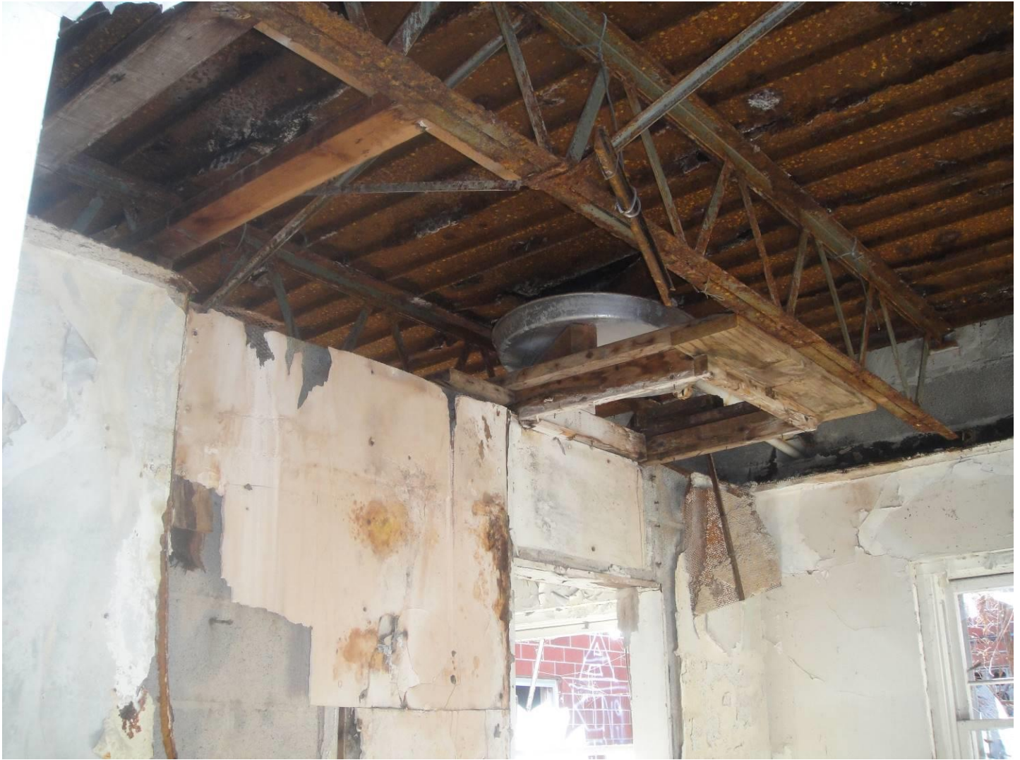
Photo 28 – Damaged/deteriorating room ceiling.
