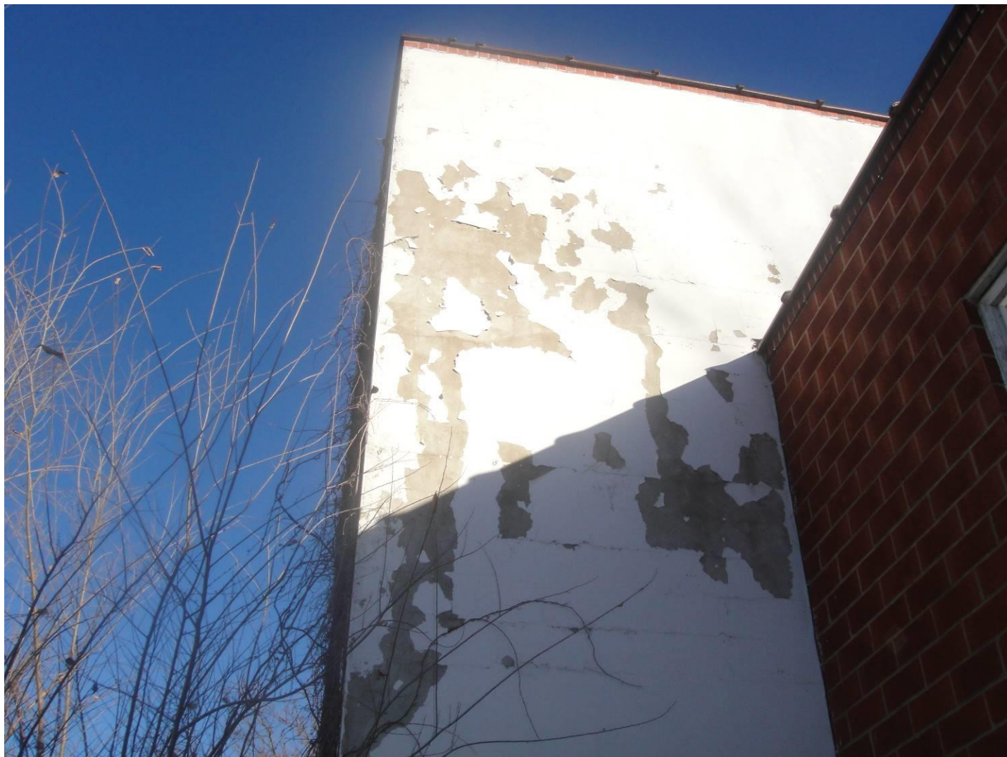
Photo 25 – Deteriorated siding material, 110 W. Main Street.
