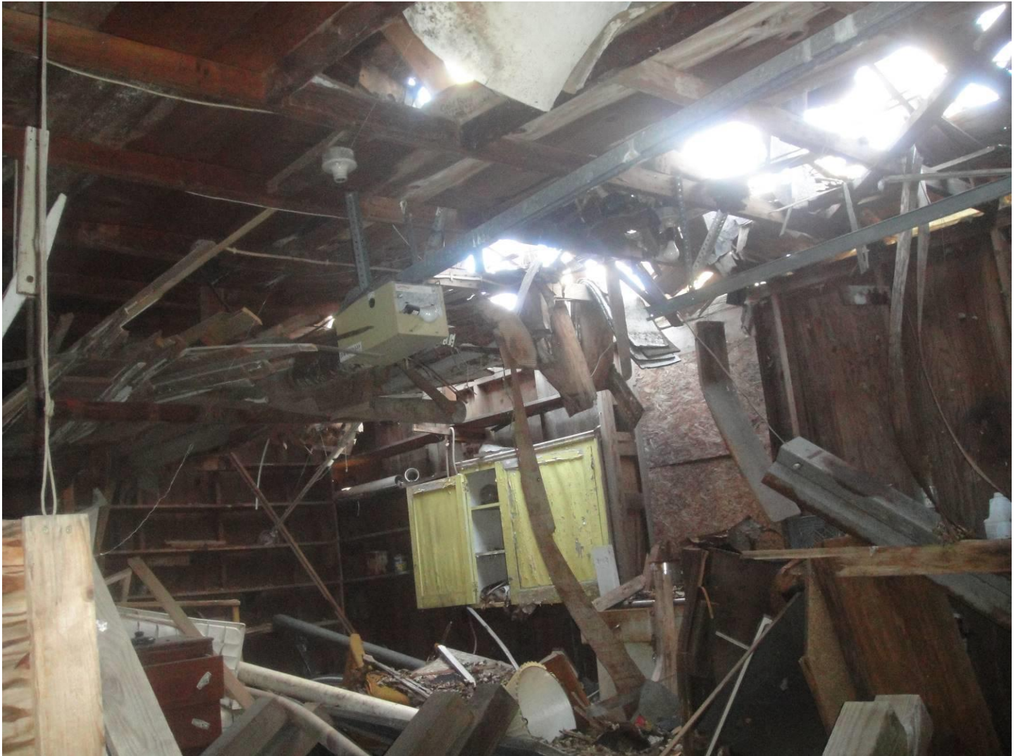
Photo 13 – View of collapsed garage ceiling.
